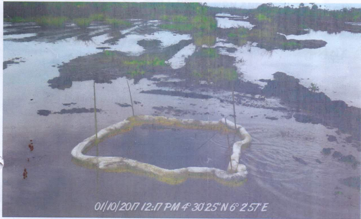
The spill point backfilled and boom used as structural control in place.
