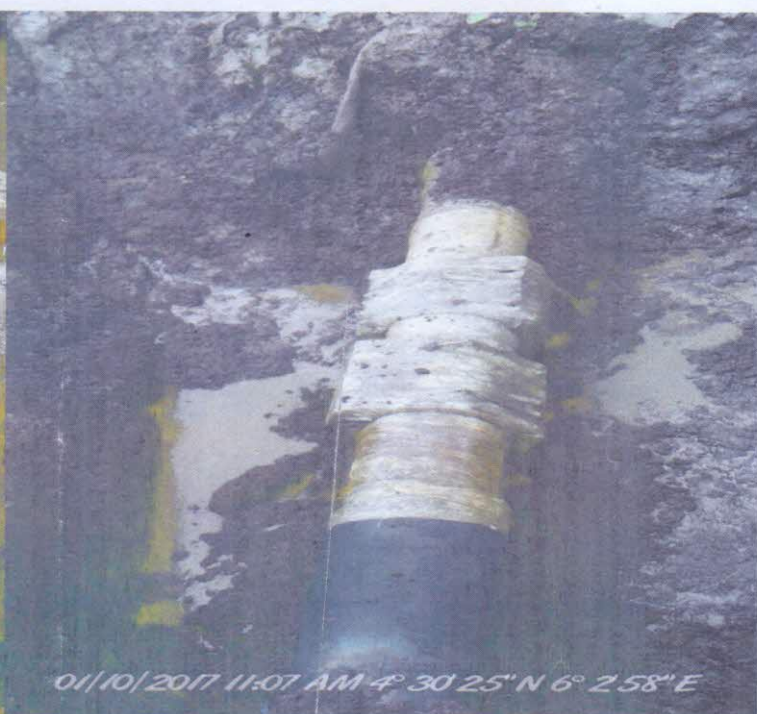
Figure 1 TWO CLAMPS SECTIONED ON THE AFFECTED PIPE LINE (1&2) AFTER EXCAVATION.
